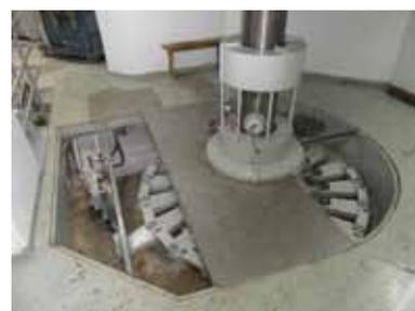
Actuation of 13 MW Turbine
